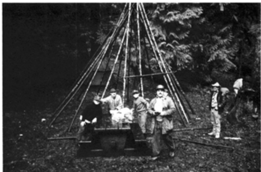
The pole frame takes shape.
